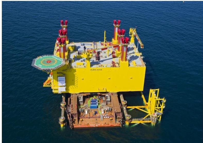
The Siemens electrical plant fitted inside the platform is capable to transmitting 864 MW into the onshore power grid making it the most powerful converter substation installed in German waters to date.
