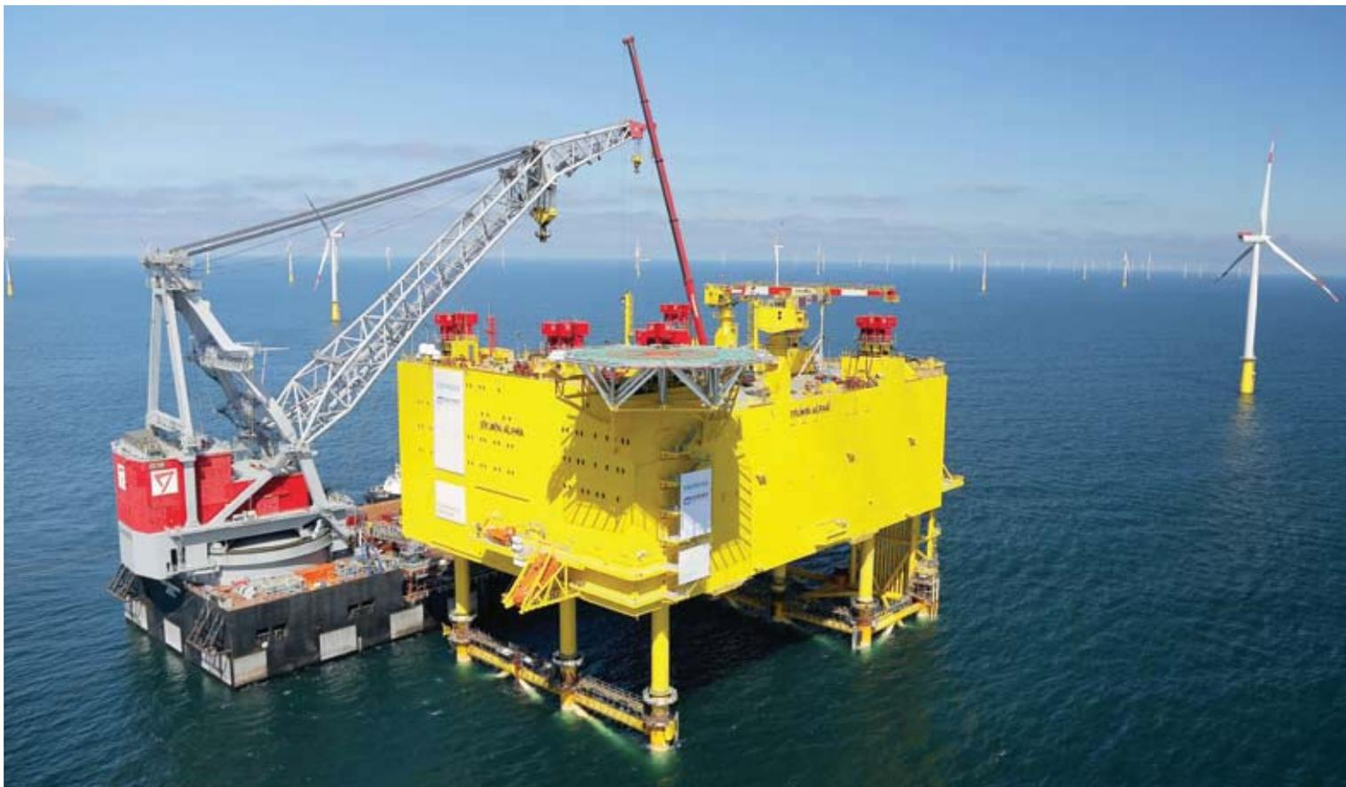
The SylWin alpha platform (864 MW) is the world's largest installed converter platform. It will transmit the energy produced by the three North Sea wind farms DanTysk, Butendiek and Sandbar ashore.
