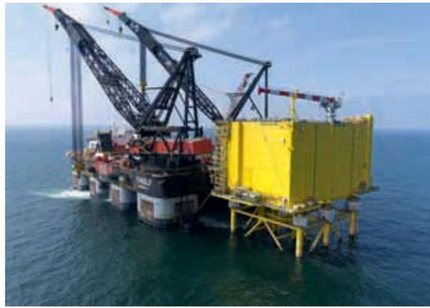
**The crane method: the topside of DolWin alpha was lifted onto the previously installed jacket by the crane vessel Thialf.**
