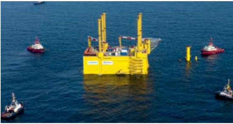
The float-over method: four tugs precisely positioned the HelWin alpha converter platform over its base frame.
