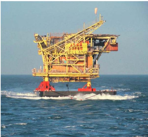
German naval architect and offshore engineering consultant Overdick was contracted as Perencos project partner for both the Welland and Sanaga projects, having earlier earned its North Sea special solution spurs with the innovative mobile offshore application barge installed alongside the existing Trent fixed production platform, also for Perenco (OE November 2005). The Welland topsides and jacket were both removed in January 2011 and transferred to shore (OE April 2011).
