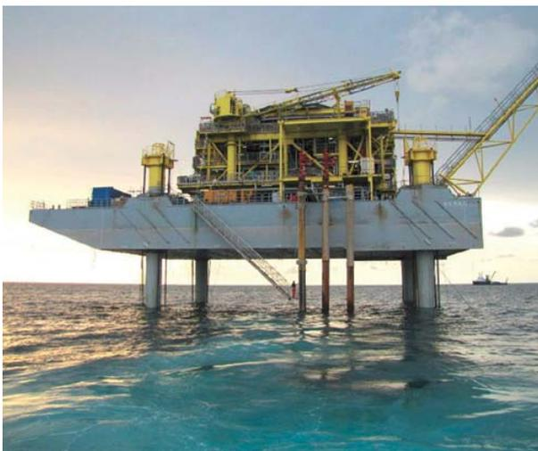
Following refurbishment by Hoondert in the Netherlands, the topsides headed for West Africa on the hull of another of Overdicks innovative self-installing leg barges. The Sanaga 01 module, with its elevated hull supporting an 1800t wellhead platform, was eventually installed in 17m of water offshore Cameroon in April this year.
