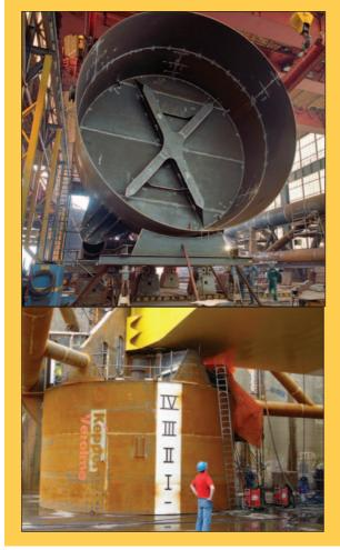
Four 9m diameter suction cans provide the seabed foundation for the barge.
