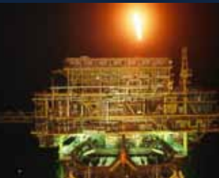
Float-overs BR-E Gas Platform
